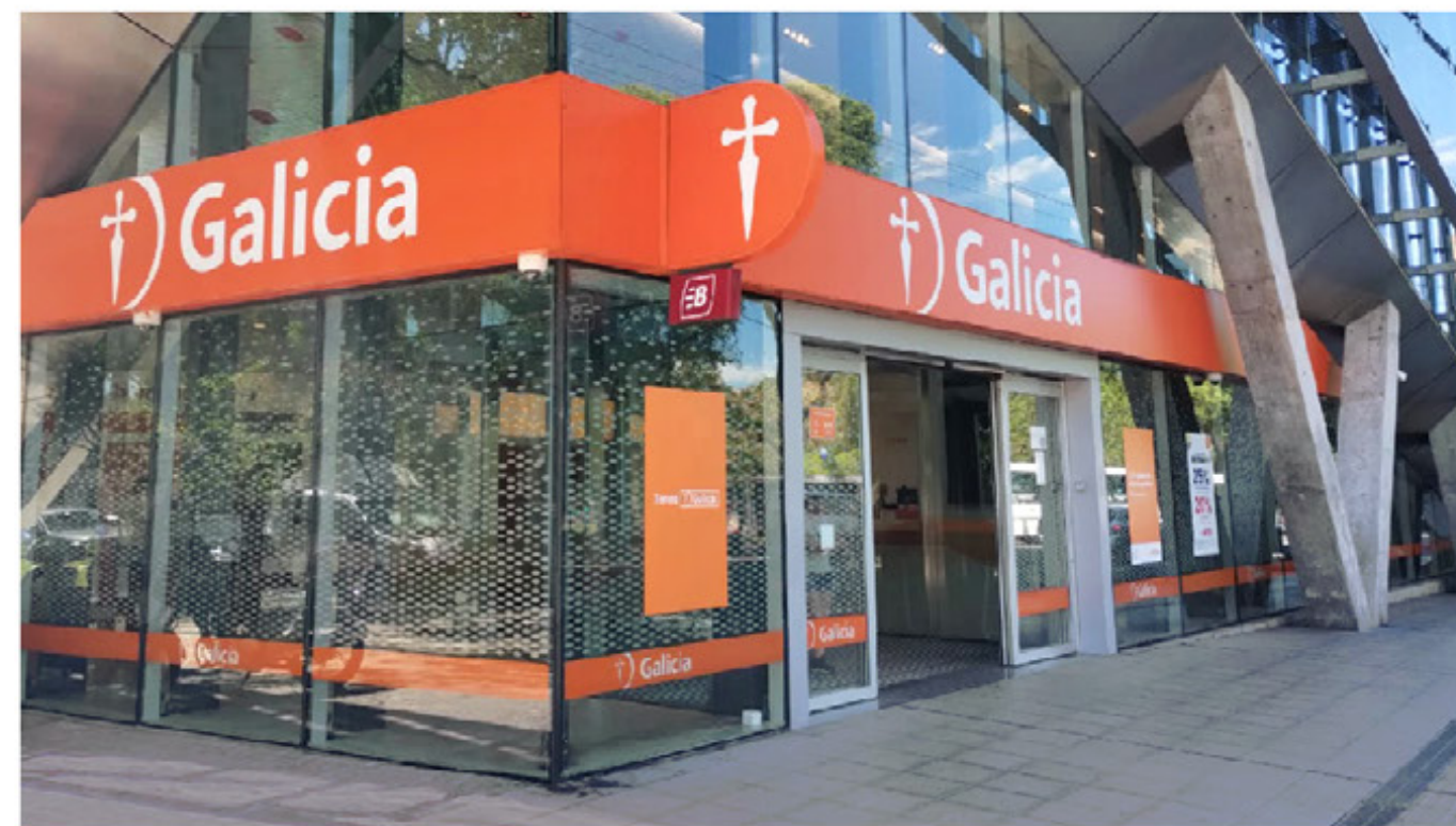
THE PLAZA GALICIA BRANCH OFFICE BECAME THE FIRST GALICIA BRANCH OFFICE TO HAVE AN ENVIRONMENTAL MANAGEMENT SYSTEM CERTIFIED UNDER THE ISO 14,001:2015
